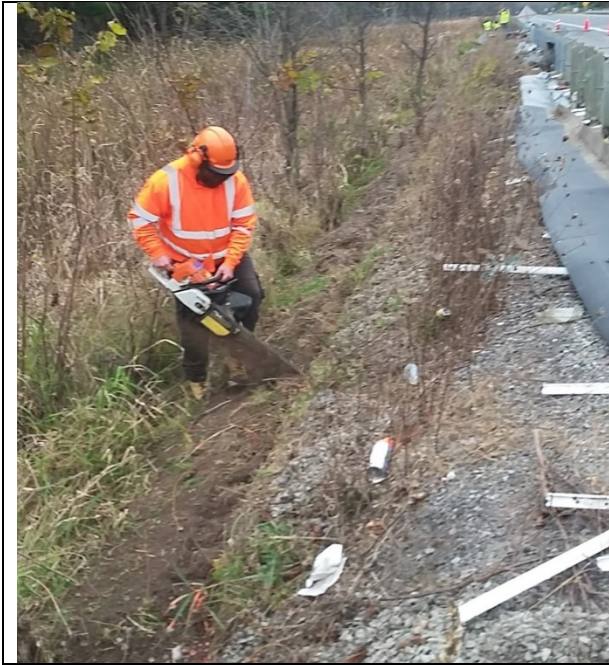
Photo 47: Preparation of ground at road slope for below-grade installation of exclusion fence, 23-Oct-18
