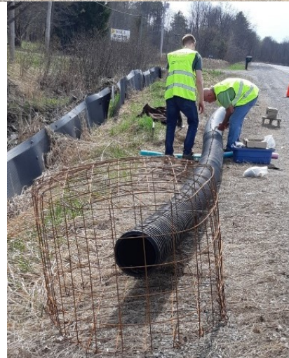
Photo 36: 6-foot 250 mm HDPE Pipe transported and assembled into protective cage on site.
