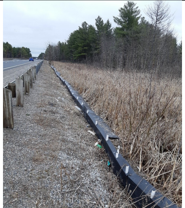
Photo 50: Viewing exclusion fence from top showing an approximate 30 cm below-grade installation (26-April-2019).
