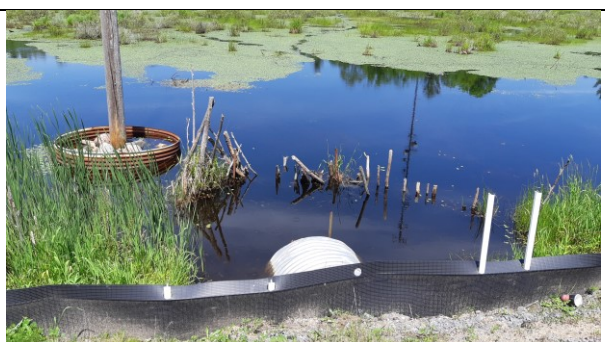
Photo 42: Exclusion fencing pulled 1 metre above north main culvert on higher ground
