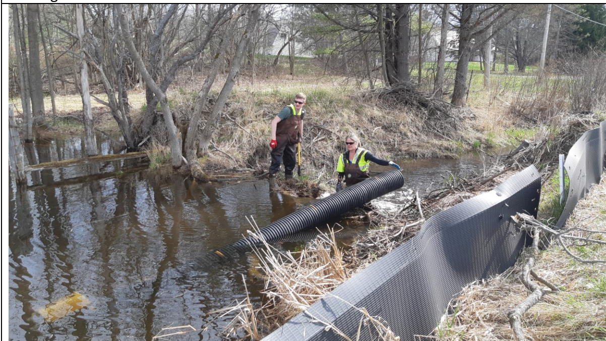
Photo 38: Placing the pipe into the beaver dam.
