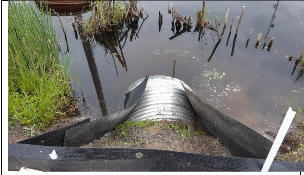
Photo 43: Guide-wall fencing extending from fence to north main culvert entrance on 13-Jun-19.
