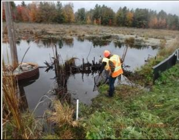
Photo 12: Construction of a diversionary dam around the north culvert entrance on Highway 7
