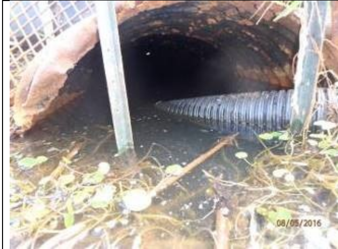
Photo 15: Culvert with two metal t-posts in front of inlet, with pipe anchored on to one (right) post for stability.
