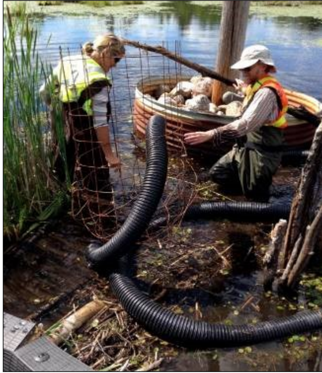
Photo 17: Implementation of cage with pipe into wetland.
