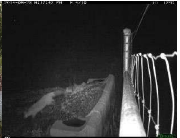
Photo 53. Gap between fence and concrete blocks
