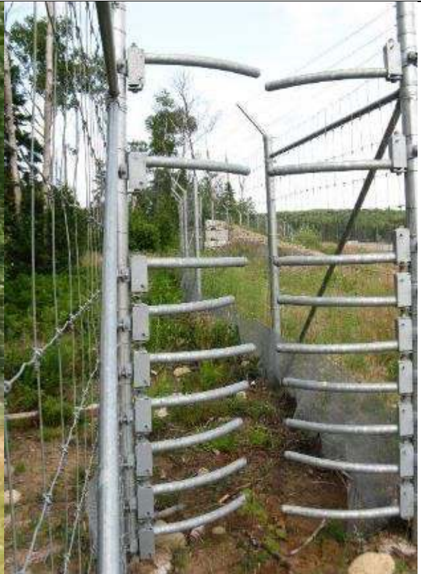
Photo 45: Zoom in of one-way gate at Sundridge with prongs open (OWW18SUN)
