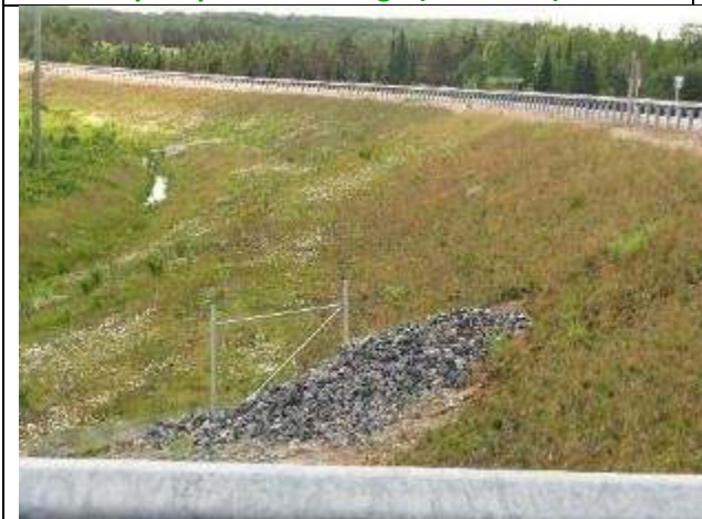
Photo 35: Highway view of rock pile treatment and moderate slope at Sundridge (FEBOUND1)
