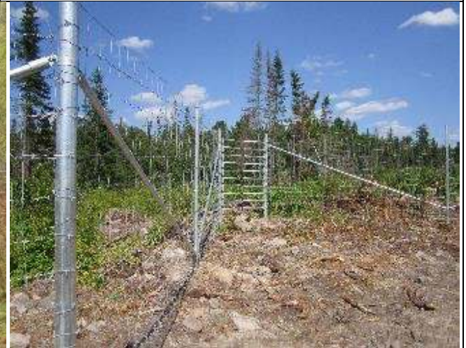
Photo 79: One-way gate installed in a V design on Highway 69
