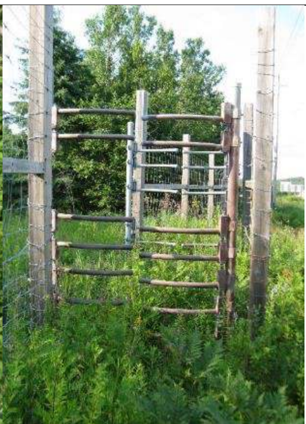
Photo 4: Paired one-way gate at Callander (second generation), 17 July 2014
