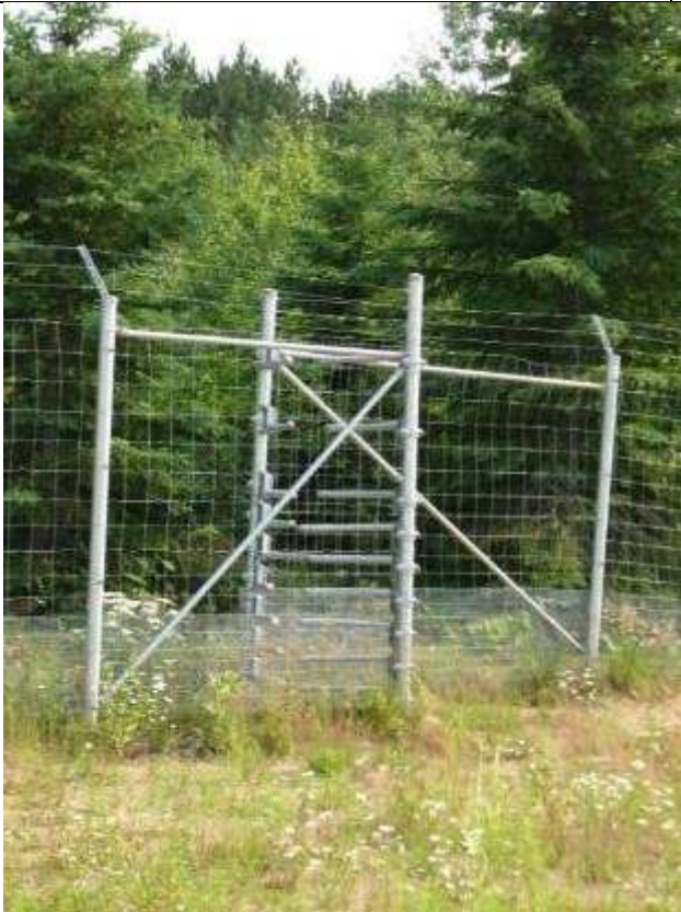
Photo 44: One-way gate with bottom apron
