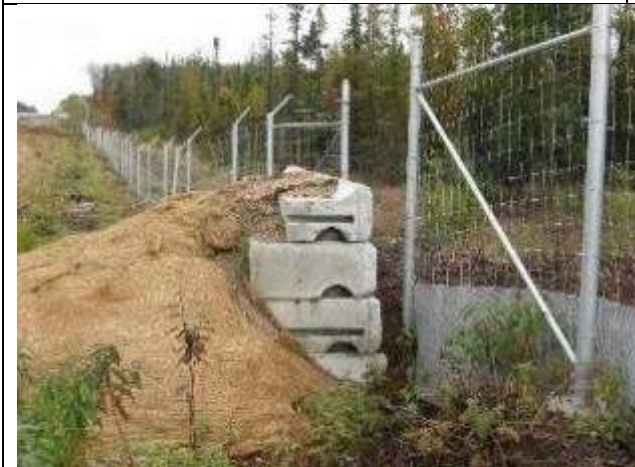
Photo 52. Jump-out side view at Sundridge with no ramp for Deer to access along fence
