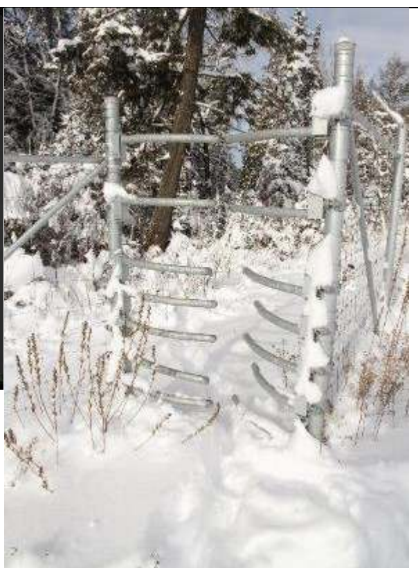
Photo 49: Deer moving through one-way gate back to safe-side (OWW12SUN) ,21 Nov-14
