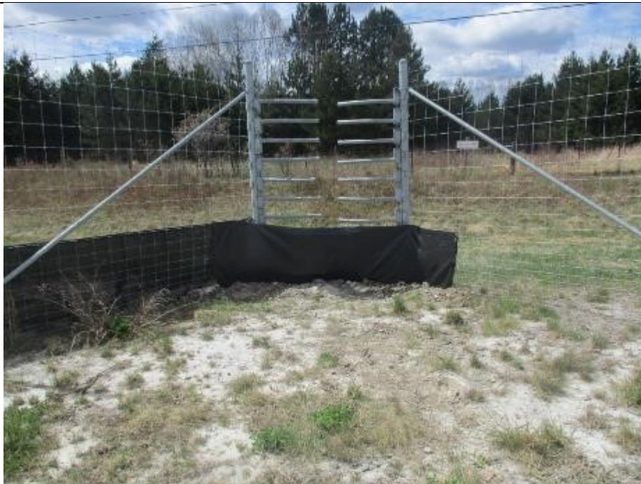
Photo 6: Closing the one-way gate between Drainage System 2 and Drainage System 3 with geotextile material (2016).
