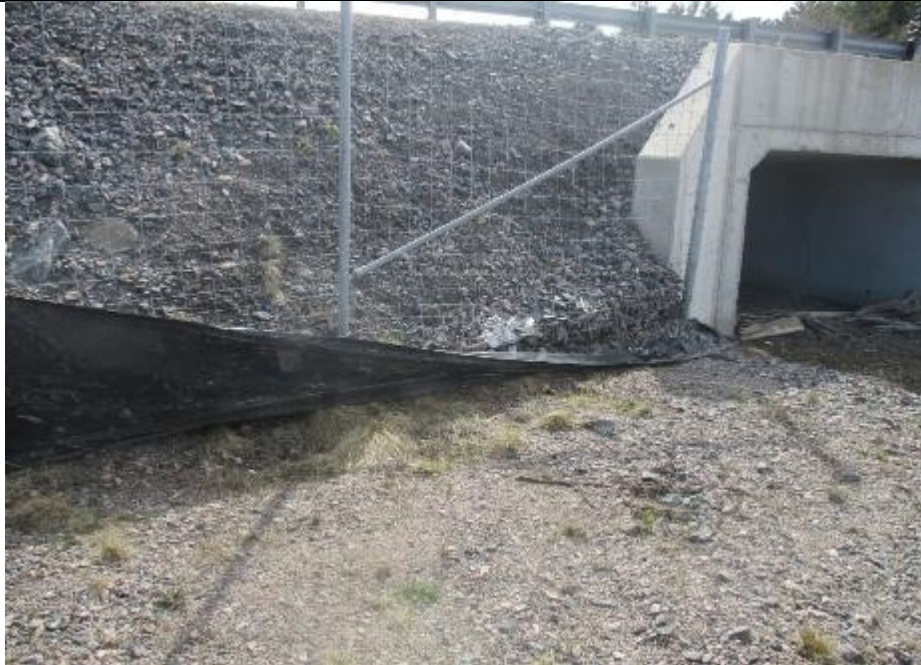
Photo 13: Fallen exclusion fencing due to rip rap erosion at the east entrance of Reptile Tunnel 2 (2016).
