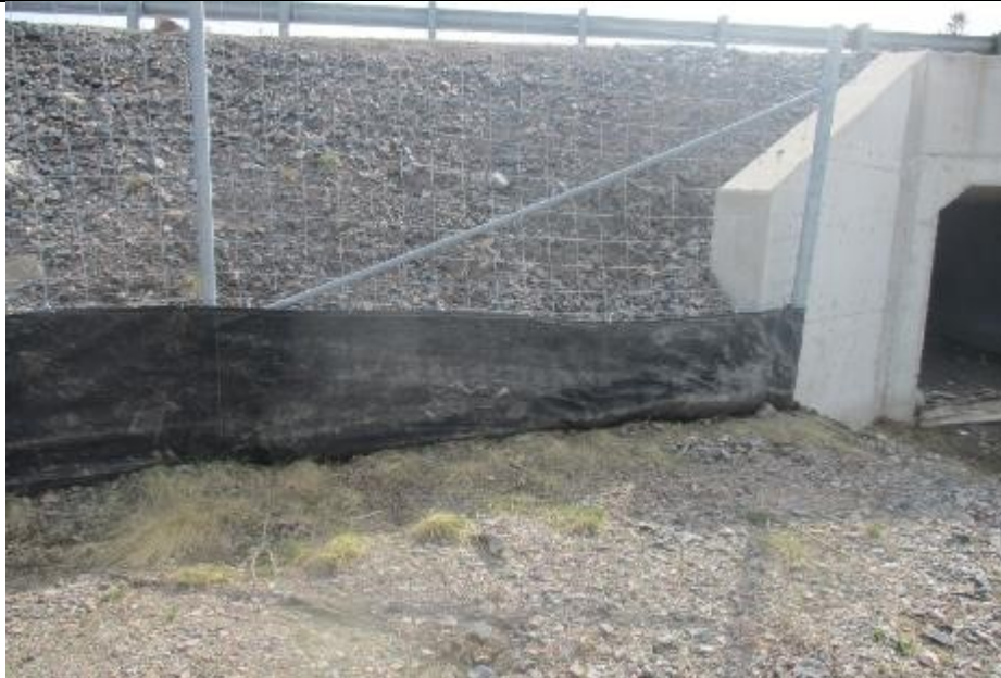
Photo 14: Repaired exclusion fencing at the east entrance of Reptile Tunnel 2 (2016).
