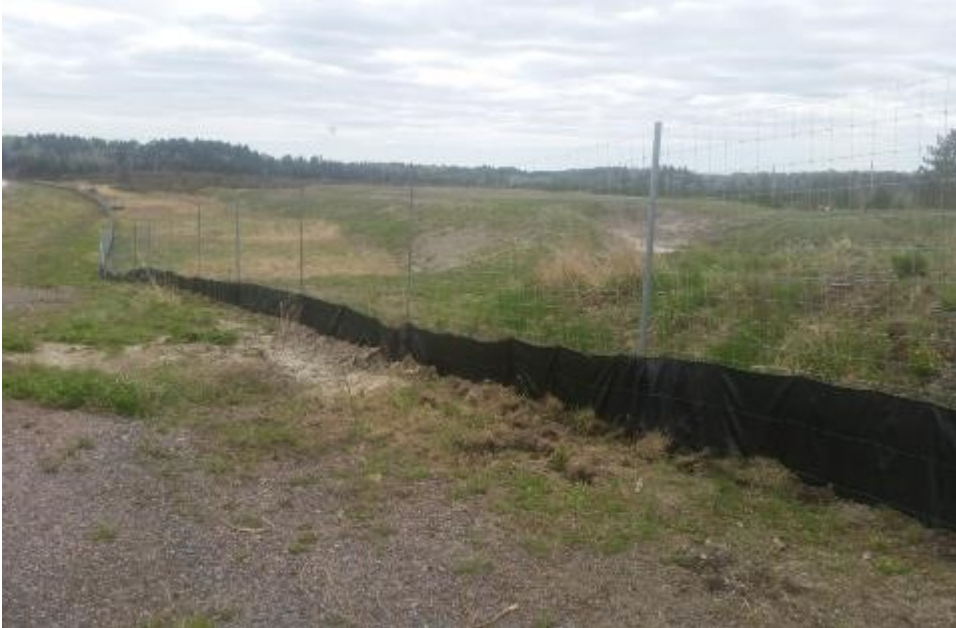
Photo 24: Reptile exclusion fencing extension on the northwest side of the highway in 2016 (19-May-2016).
