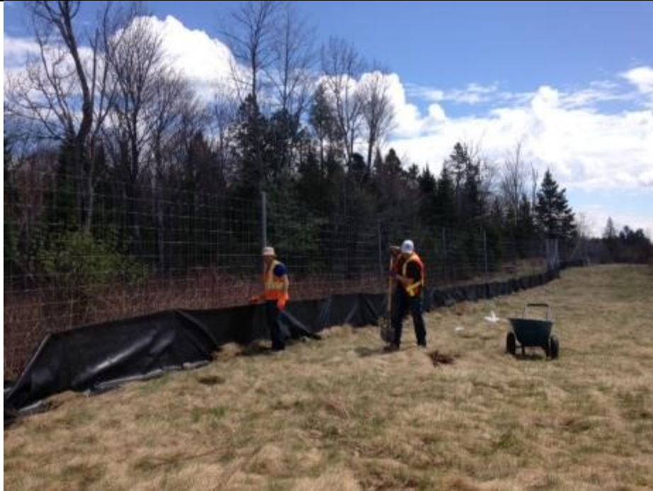
Photo 19: Installing reptile exclusion fencing on the east side of Highway 69, at the south end of the Sheppard Lake transect (13-May-16).
