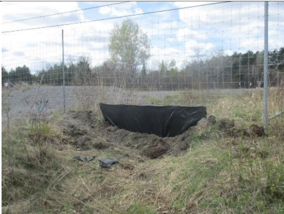
Photo 4: A five meter piece of geotextile material installed in 2016 to close the gap under the fencing between Drainage System 2 and Drainage System 3.
