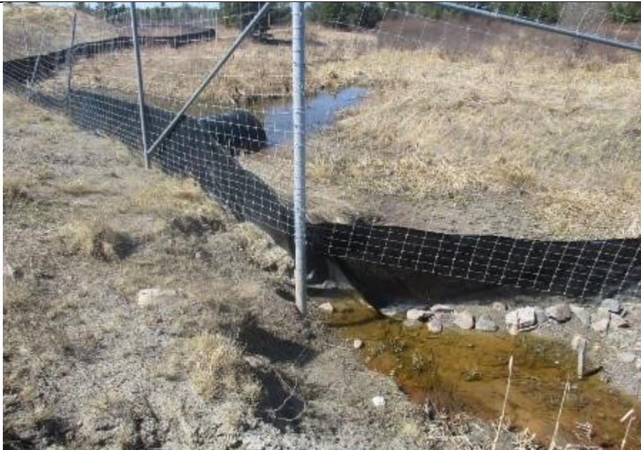
Photo 1: Drainage System 1 west end washout prior to repairs in 2016. This section of fencing also experienced a washout in 2015.
