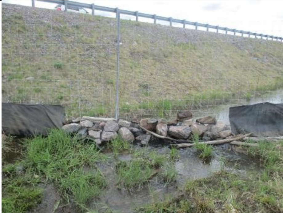
Photo 12: Zoom-in of rock wall that permits water flow built in 2015 and repaired in 2016, at the east entrance of Reptile Tunnel 1.
