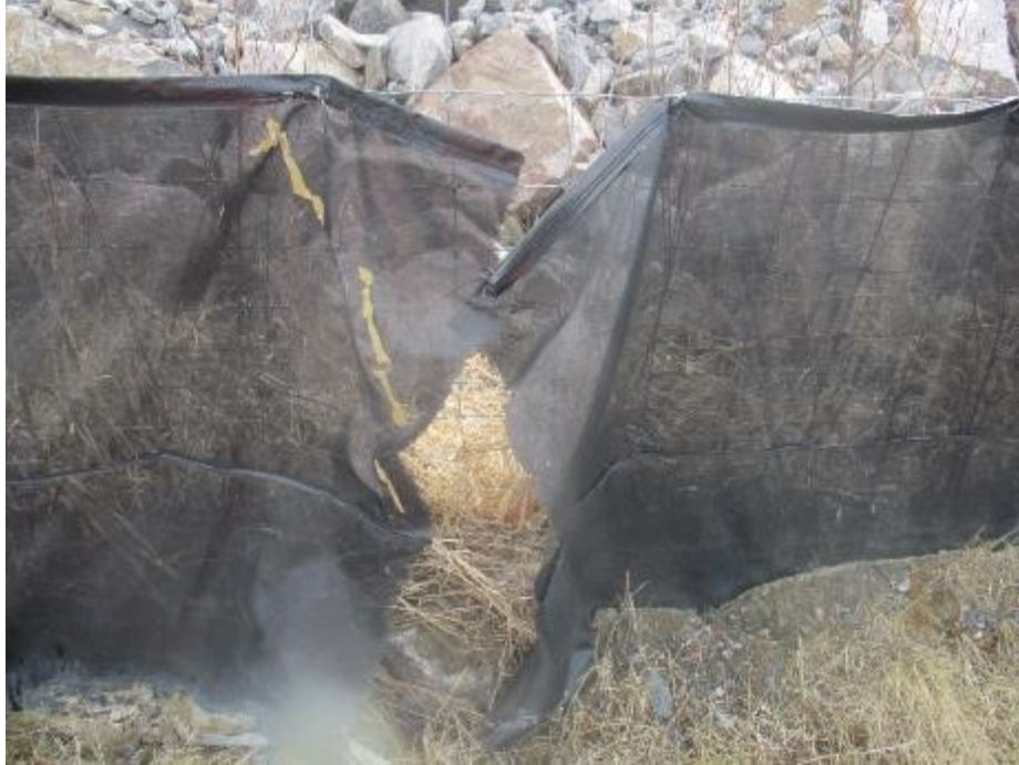
Photo 7: A rip in the reptile exclusion fencing on the west side of Highway 69 between Reptile Tunnel 1 and the northwest fence end (2016).
