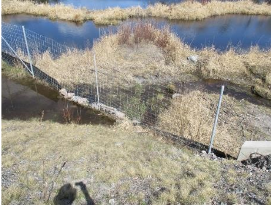
Photo 11: Change in hydrology at the Reptile Tunnel 1 east entrance. Water had flattened the reptile exclusion fencing in 2015. Fence was cut and rocks were used as barrier to exclude turtles but allow water flow, this was maintained in 2016.
