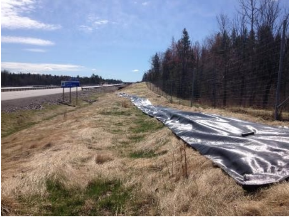
Photo 17: Installing reptile exclusion fencing at the south-west side of Sheppard Lake transect (9-May-16).
