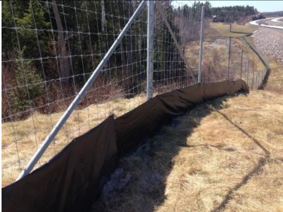
Photo 18: Installing reptile exclusion fencing at the south-west side of Sheppard Lake transect (10-May-16).
