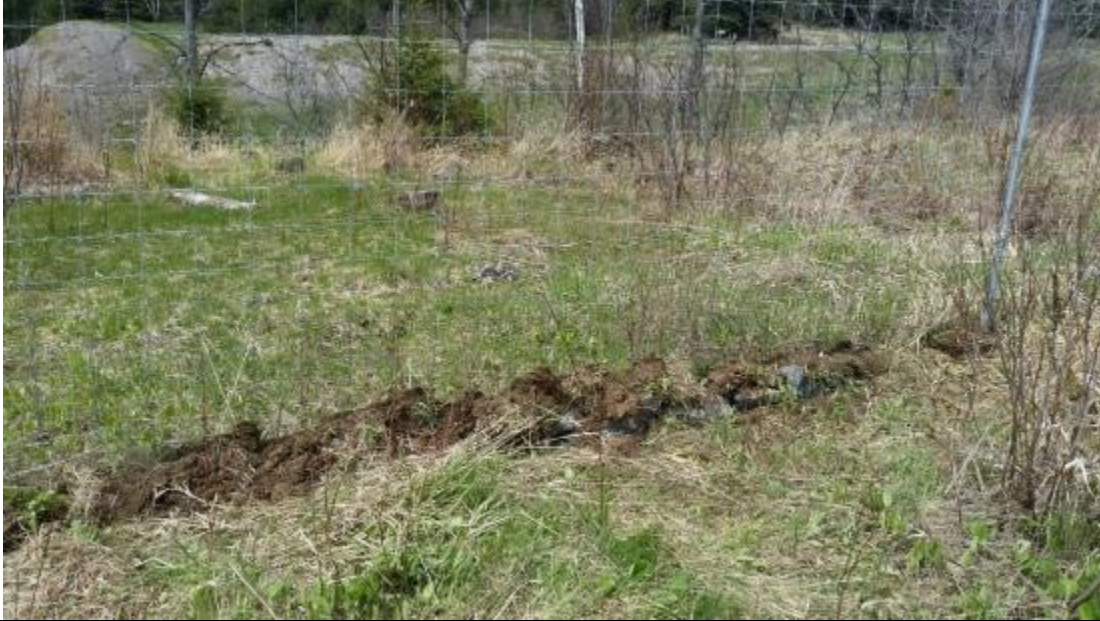
Photo 23: Rocks and dirt used to fill gaps at bottom of fence at northwest fence extension (16-May-2016).
