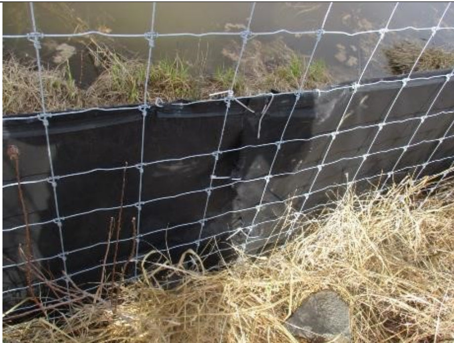
Photo 10: Second rip repaired between Reptile Tunnel 1 and the northwest fence end (2016).
