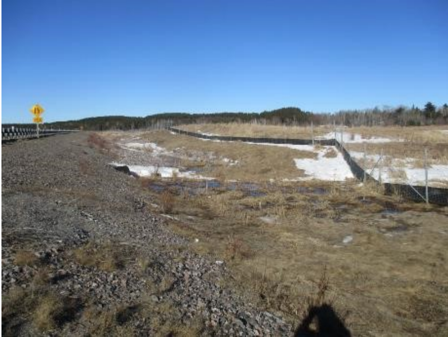
Photo 15: Non-functional drainage culvert (DS1) for wildlife passage because east end not extending through wildlife fencing.
