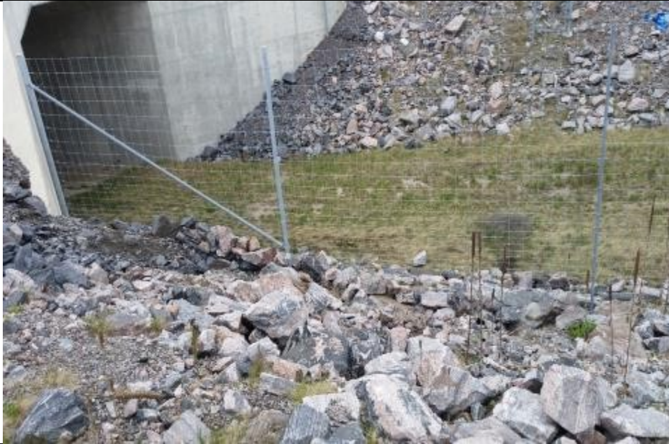
Photo 21: Large rocks stacked along the bottom of the fence to close gaps in the large animal underpass median (2016).
