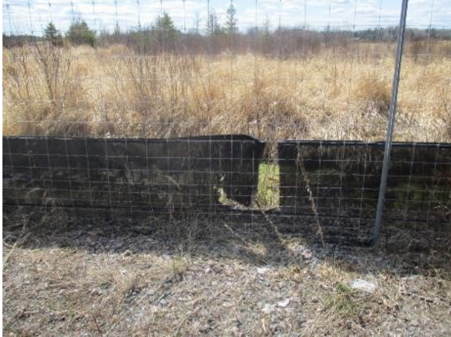
Photo 9: A second rip in the reptile exclusion fencing on the west side of Highway 69, between Reptile Tunnel 1 and the northwest fence end.
