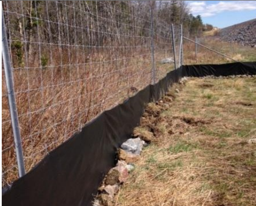
Photo 20: Completed reptile exclusion fencing at the east side of the large animal underpass; this location was the end of the Sheppard Lake transect in 2016.
