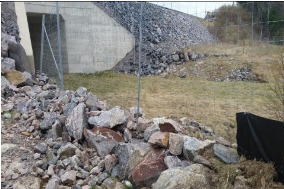
Photo 22: Reptile exclusion fencing extending to the west side of the large animal underpass (2016).
